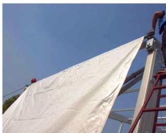
Roof Fabric Installation
